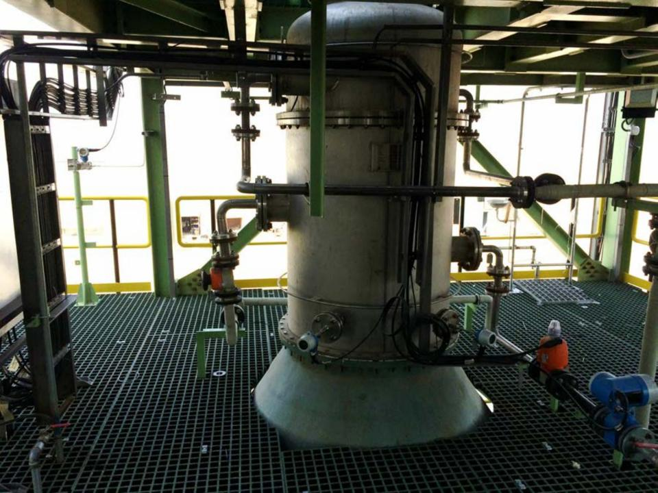
**Variable throat venturi** To remove SO<sub>3</sub> aerosols and any residual antimony oxide dust
