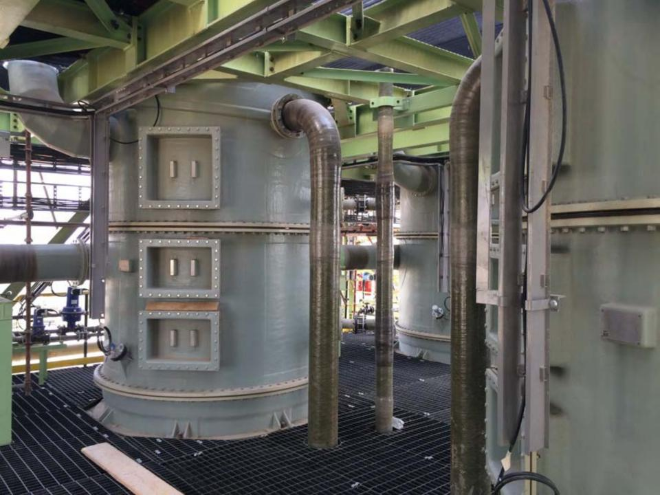
**Top of GRP lined V-tex® sump tank** V-tex® scrubber reaction and oxidation tank, scrubbing liquor reservoir and feed tank to gypsum dewatering Epoxy lined steel tank, fabricated *in situ*
