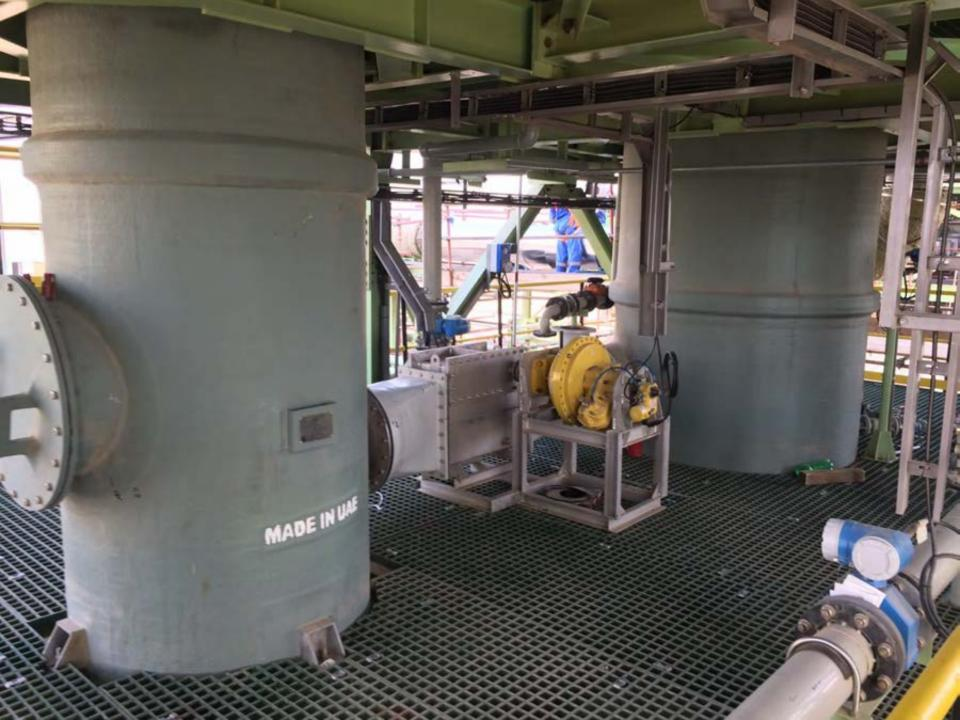
Acid circuit pump skid assembled at ERG PF Supplies scrub liquor to the quench, sub-cooler and venturi, runs on 10% sulphuric acid PP pumps and pipework
